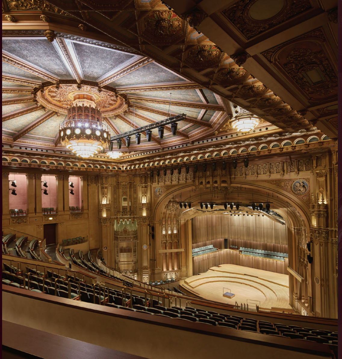
Historic fixtures were refurbished to incorporate modern light sources. The central chandelier's deceptively large support includes multiple layers of internal illumination and ceiling uplight.
