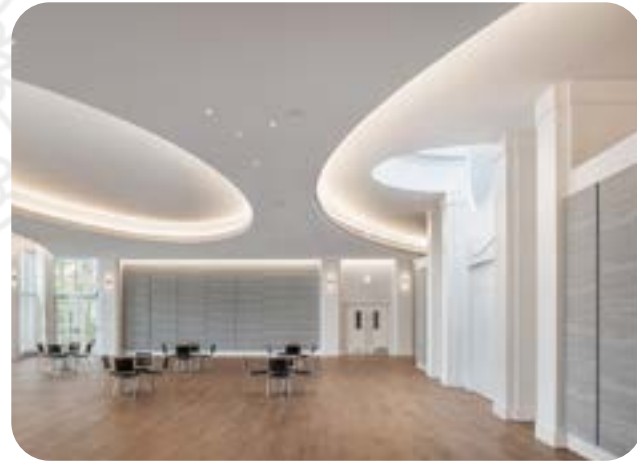
The elongated curved coves fill the space with indirect illumination while complementing the existing architectural façade, visible through the window.
