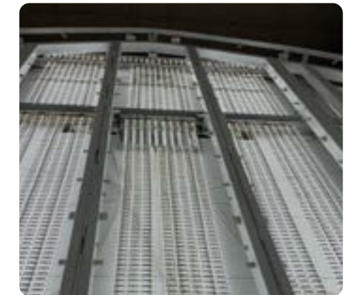
Tension-cable LEDs suspended 4.5" behind the stained-glass, delivering approximately 1,330 lumens/sq.ft. of area. Double-sided LED boards face the stained-glass and a highly-reflective matte-white surface.
