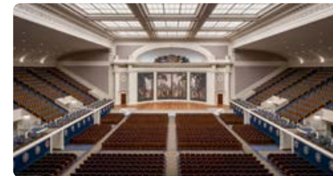
An array of 972 edge-lit LED fixtures are custom fit within the existing laylight framing to mimic the diffuse daylight seen in historic photographs.
