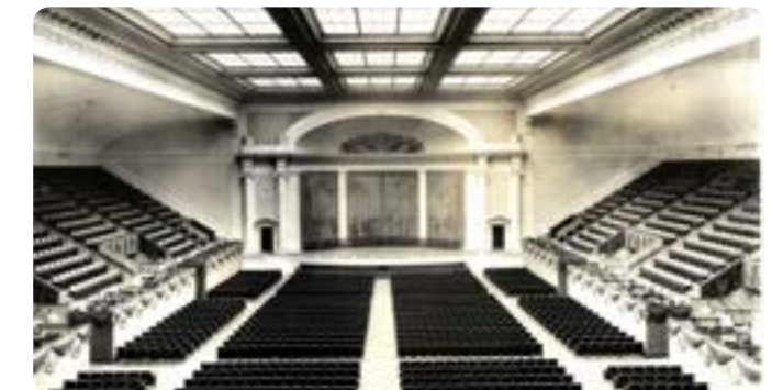
An expansive central laylight originally flooded the room with daylight. An operable 'Ventilighter' louver system in the attic provided control of the intensity for performances.
