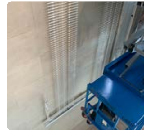
Rolling-frames deployed for maintenance, showing white "umbilical power cords" disconnected to allow retracting the frame from both sides. All junction boxes were painted matte white.
