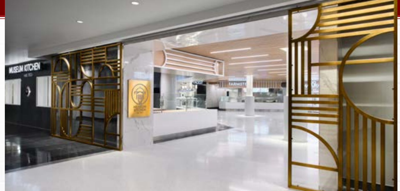
New LED downlights increase general light levels at entrance and welcome visitors into the Museum Kitchen. When open, gates are highlighted from cove-mounted linear LEDs.
