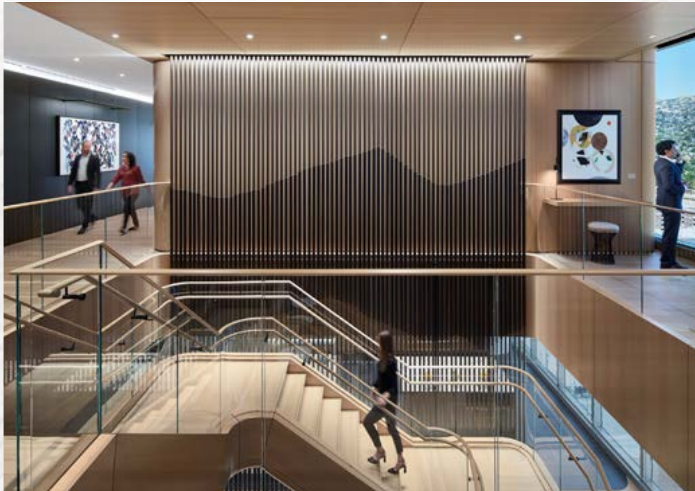
An open, 4-story stair is the primary feature of this new office. Vertical “rods” that mimic mountain ranges are illuminated by carefully-integrated linear “grazers”.
