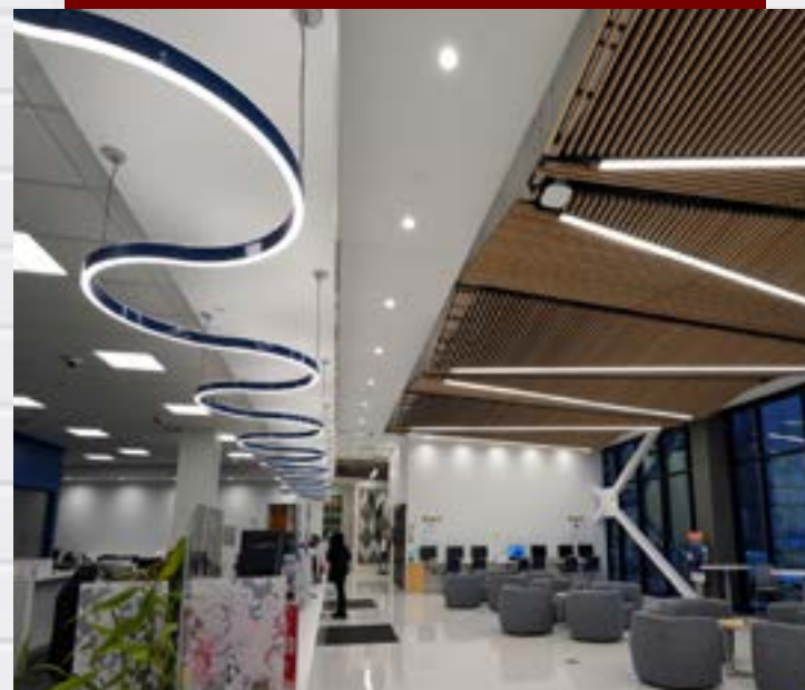
Space programming and space activities were clearly delineated by utilizing unique lighting design solutions and fixture types, while providing a harmonious symbiotic space.
