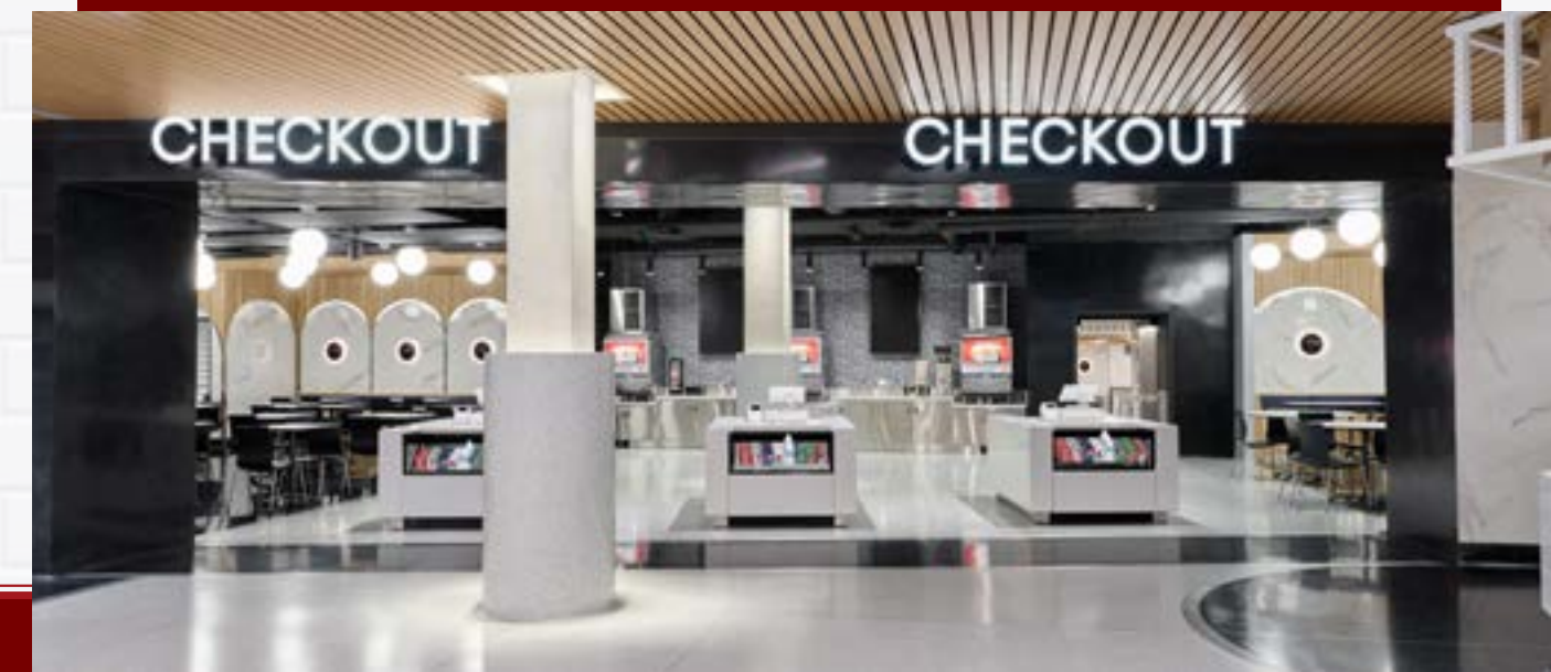
Illuminated "Checkout" signage directs guests to transaction counters highlighted by simple Unistrut-mounted cylinder adjustable downlights. Beverage station beyond is similarly illuminated by Unistrut-mounted cylinder wallwashers.
